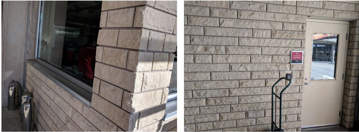
Figure AF-2: Stone Veneer Wall Location: Plaza Level 3 – 03.54.02 Security & Fire Command
