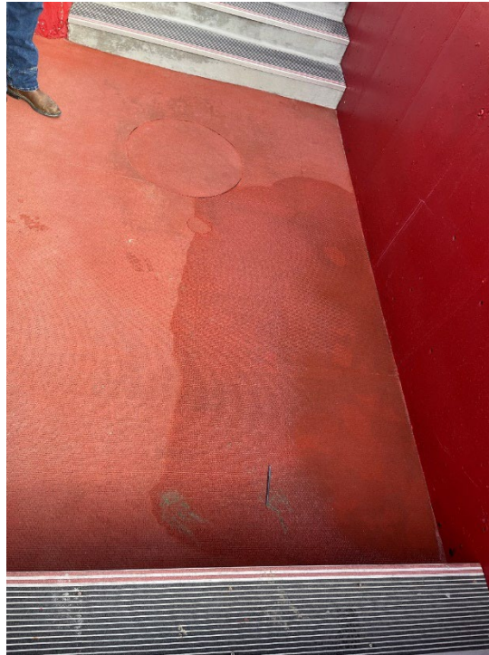
Figure C-8.1: Wet Walking Area Location: Adjacent To Chief's Locker Room Tunnel
