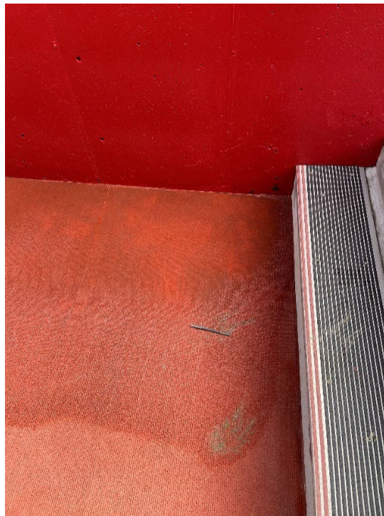
Figure C-8.2: Wet Walking Area Location: Adjacent To Chief's Locker Room Tunnel
