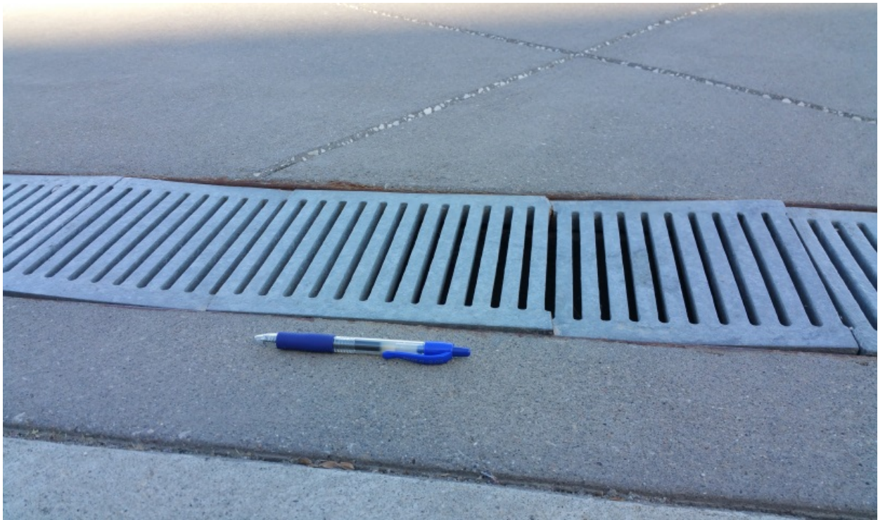
Figure C-6: Broken Trench Drain Grate Observed near Founders Plaza
