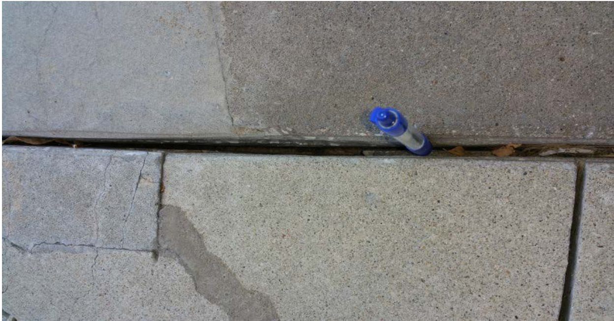
Figure C-5: Missing Sealant at the Isolation Joint near the Hy-Vee Gate
