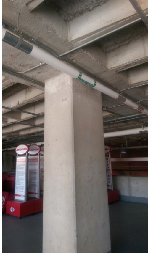
Figure S-2: CIP Reinforced Column with Pan Joist Slab System
