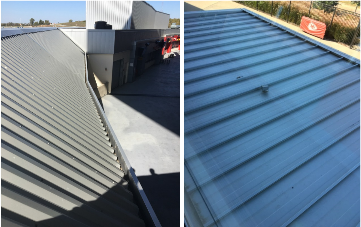
Figure AR-2: Standing Seam Metal Roof Panels
