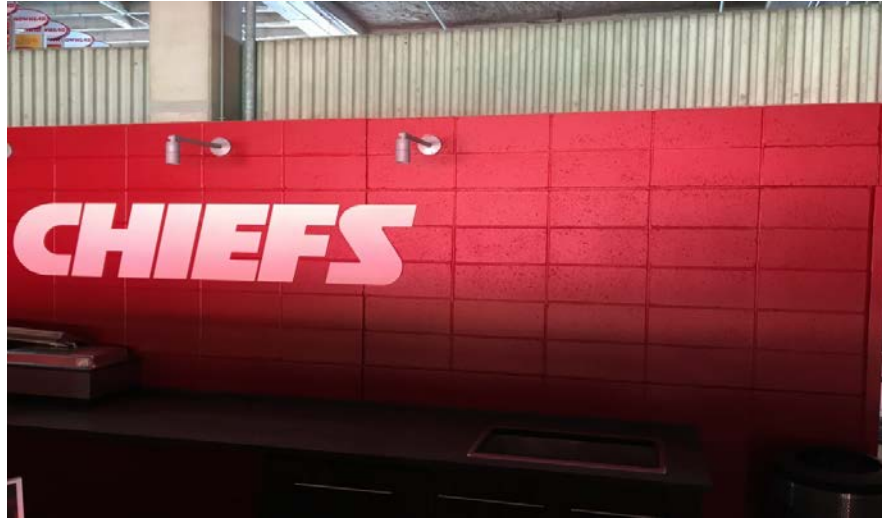
Figure AI-3: Painted, Exposed CMU Block Wall
