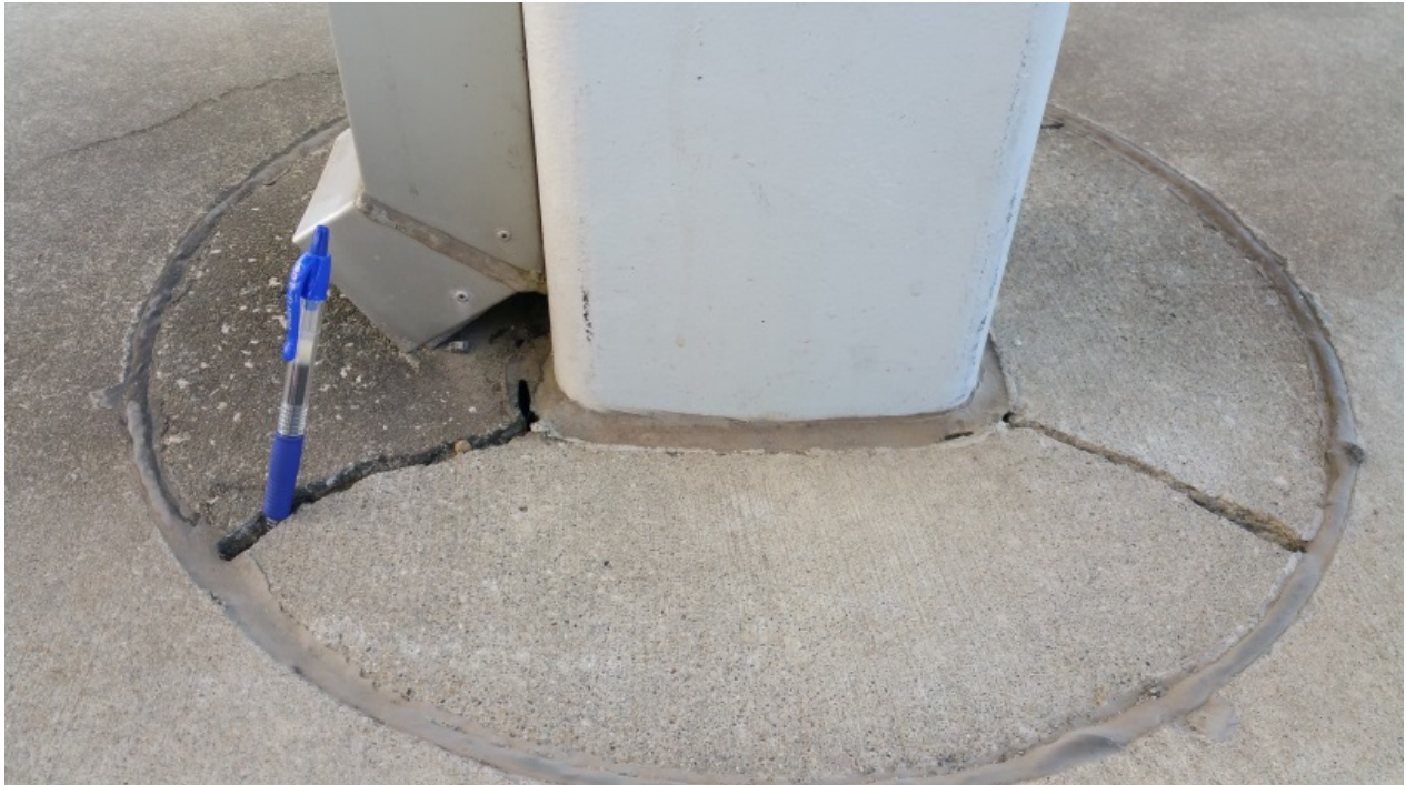
Figure C-10: Cracking at a Column Base near Gate D
