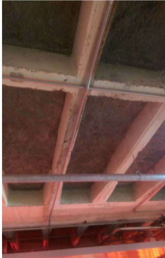
Figure S-4: Pan Joist Slab System Showing Minor Cracking
