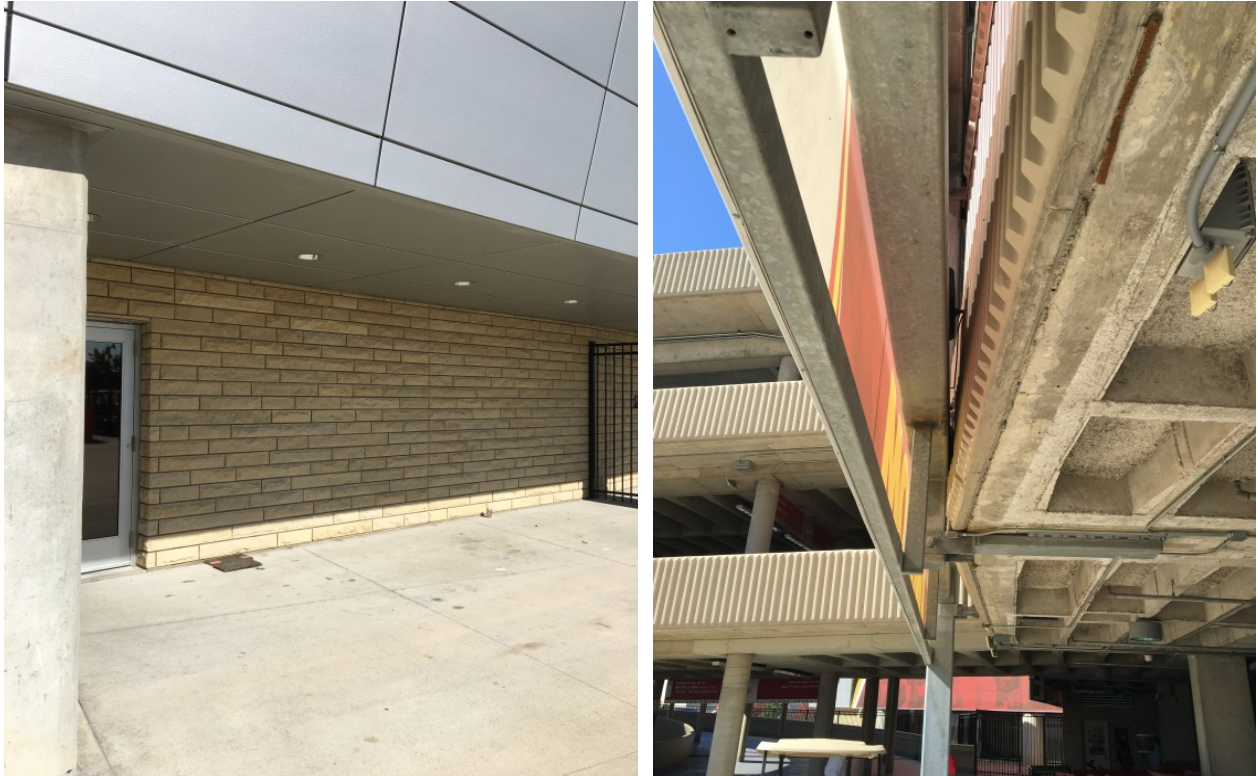
Figure AF-3: Stone Veneer Wall (left) and Graphic Fabric Mesh System (right)
