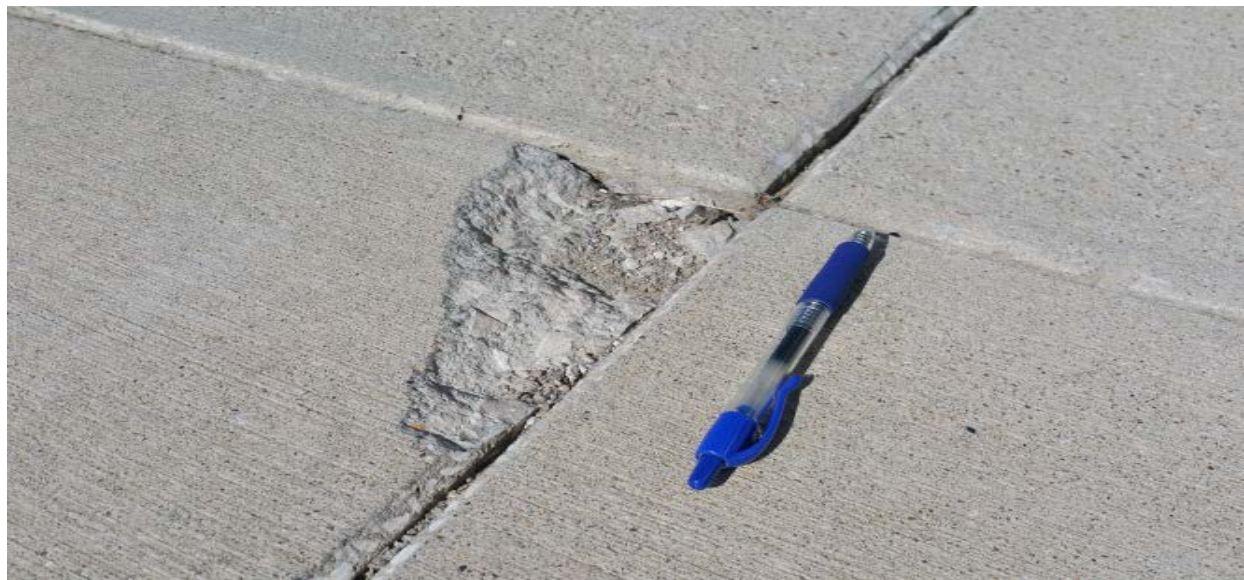
Figure C-4: Corner Spall and Cracking
