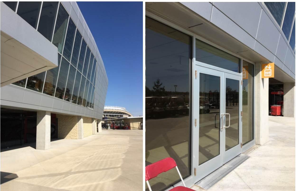
Figure AF-2: External Glass Curtainwalls and Storefronts
