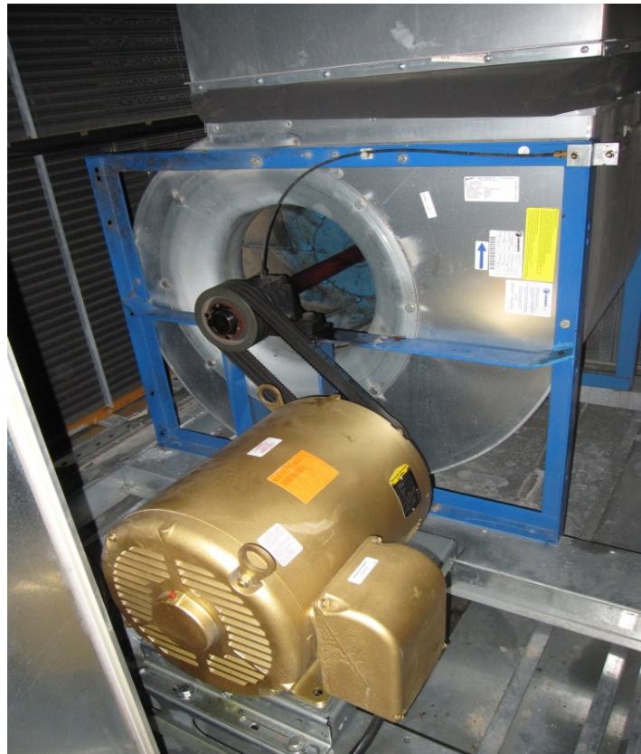
Figure M-2: AHU Fan and Motor
