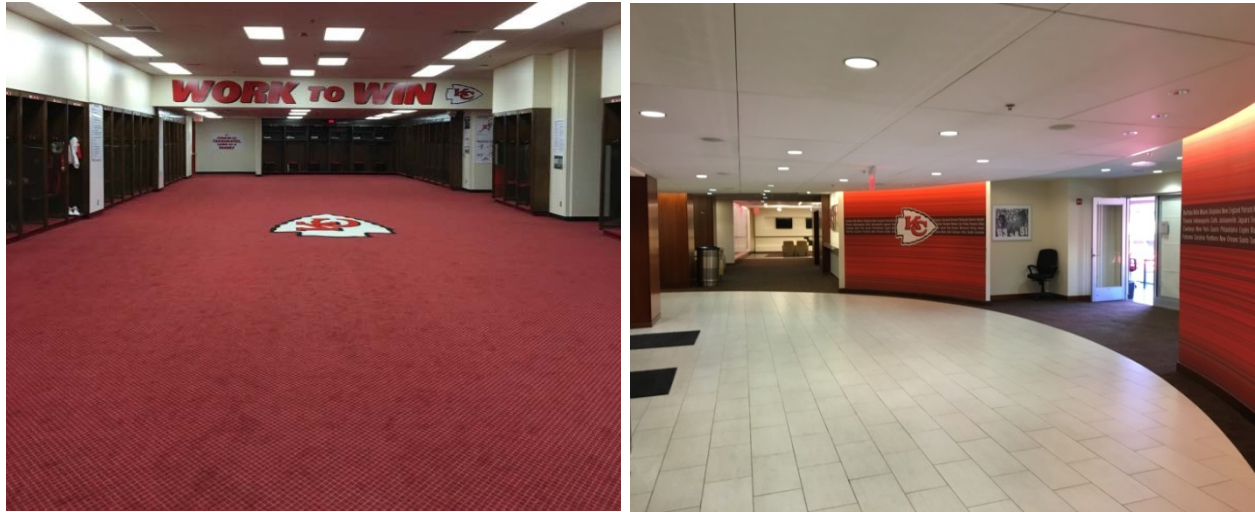
Figure AI-2: Carpet Flooring (left) and Porcelain Tile Flooring (right)
