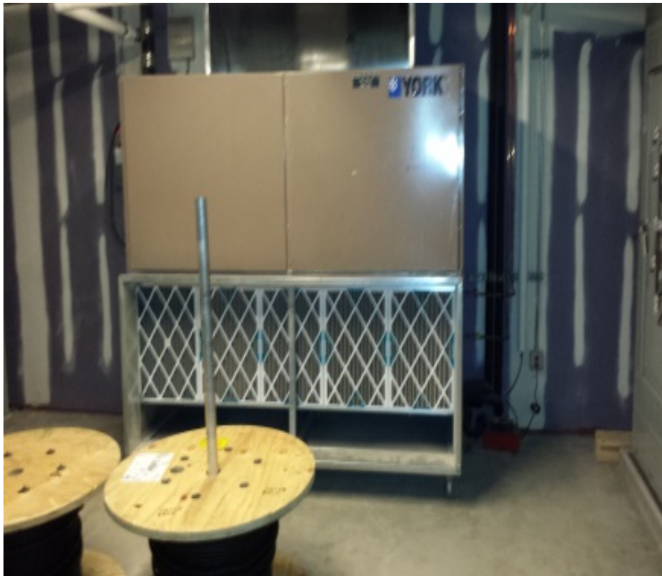
Figure M-1: Electrical Room Vertical Air-Conditioning Unit
