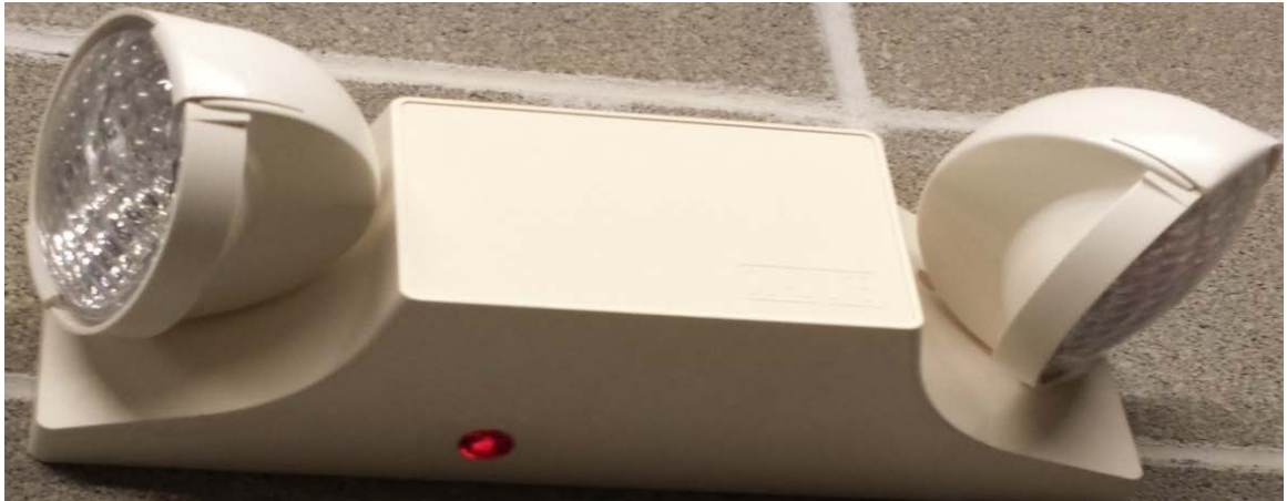
Figure E-2: Emergency Bug-Eyed Light Fixture
