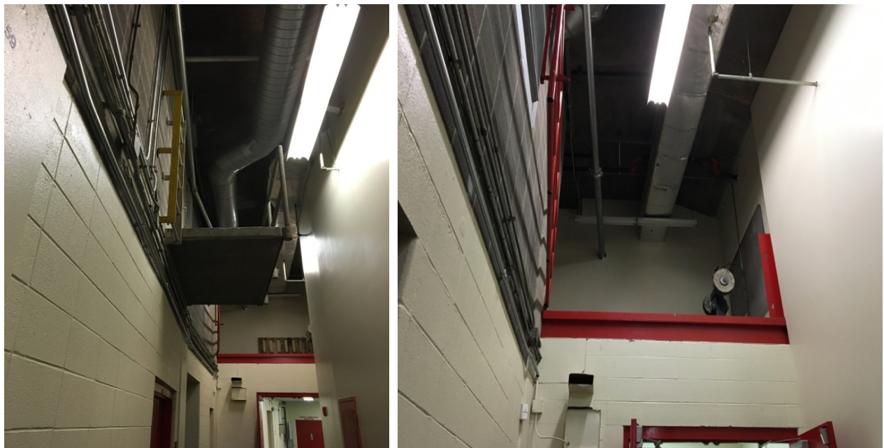
Figure AI-9: Balcony Areas without Proper Fall Protection
