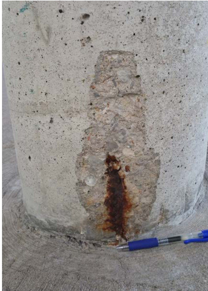
Figure C-9: Exposed Rebar within Column
