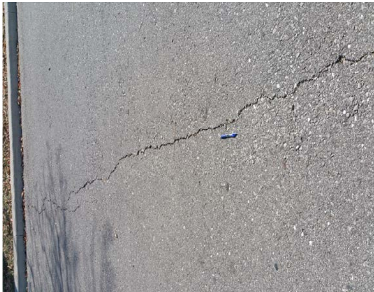
Figure C-1: Transverse Crack
