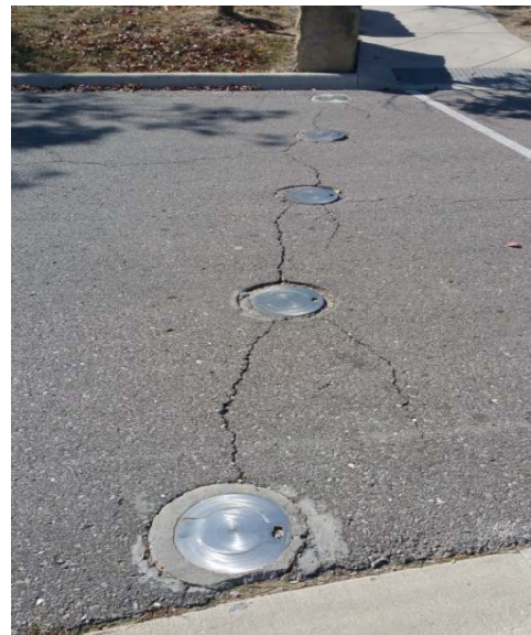
Figure C-2: Transverse Cracking at Bollards
