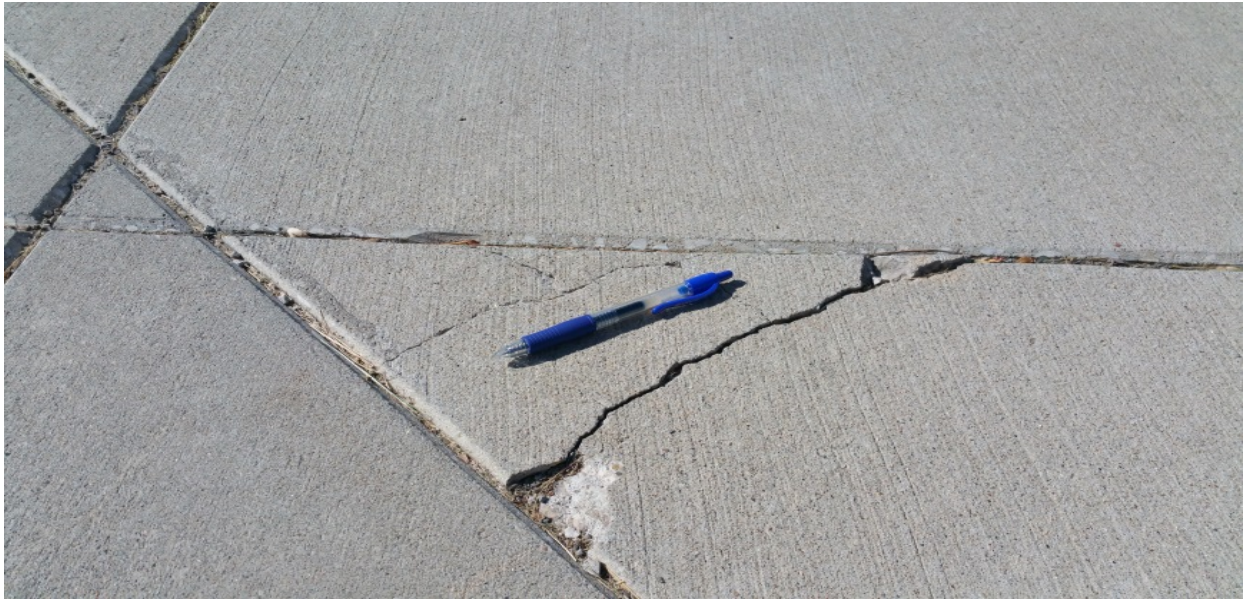
Figure C-3: Corner Spall Observed near Tower Gate
