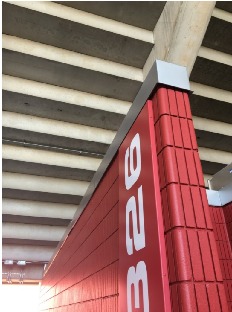
Figure AR-1: Typical Prefinished Metal Coping at Concourse
