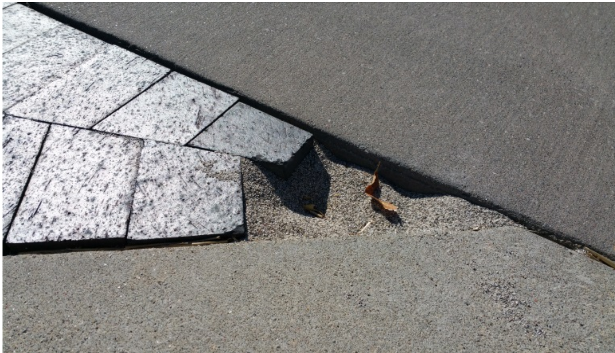
Figure C-7: Missing Paver in Main Pedestrian thoroughfare at Founder's Plaza
