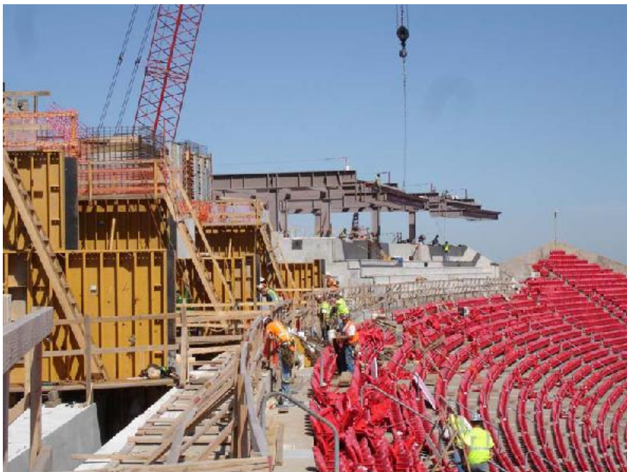
Steel Installation-Horizon Level
