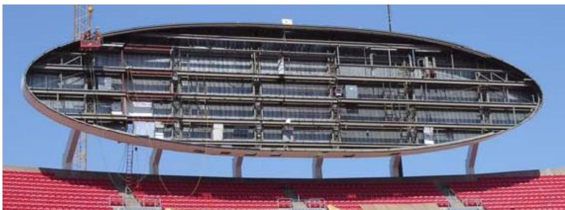
Prep work begins on West Endzone Scoreboard
